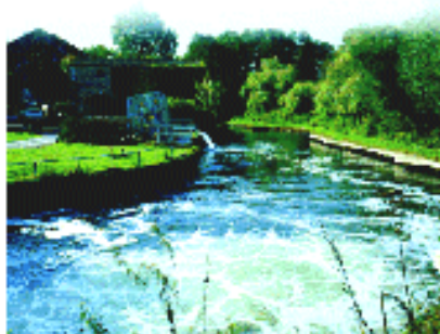
Gaters Mill intake on the River Itchen
