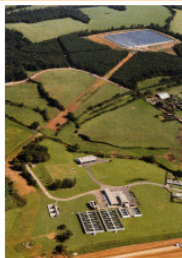
Highwood Reservoir and Itchen Treatment Works
