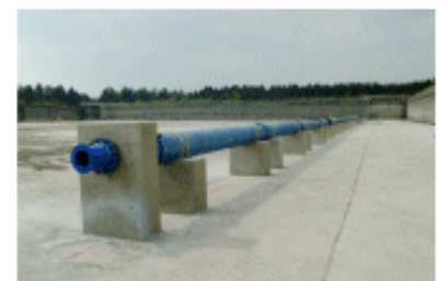
Highwood raw water storage reservoir
